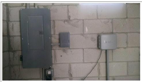
There is an electric panel for power to the storage room and pool pumps and heater inside the room.
